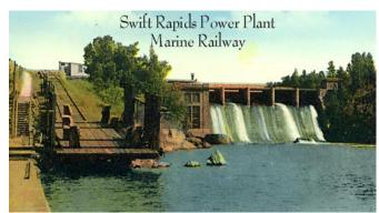
The new power plant at Swift Rapids had a capacity of 6000 horsepower at a total cost of more than \$150,000. The marine railway opened up navigation for boats through the new Trent-Severn Waterway connecting Lake Ontario to Lake Huron.
